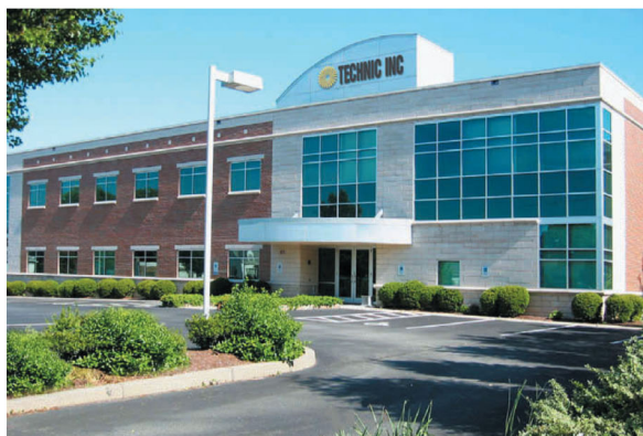
Technic Corporate Headquarters, Cranston, RI USA
